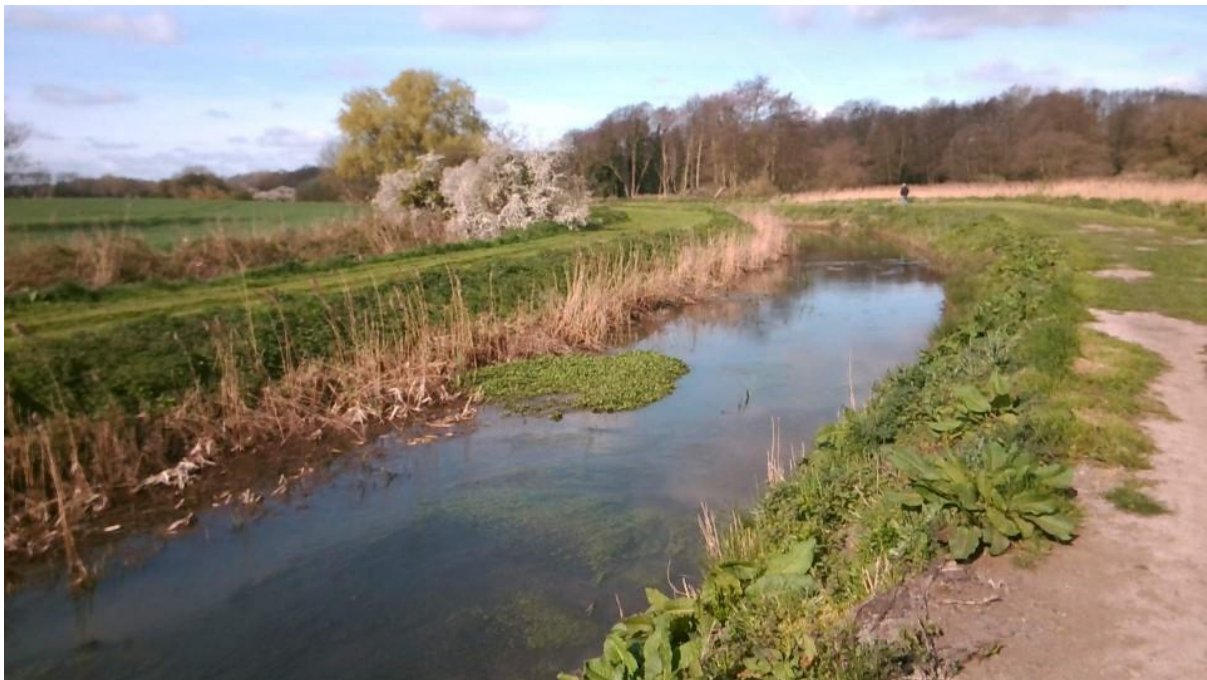
Plate 3.1 North Walsham and Dilham Canal
